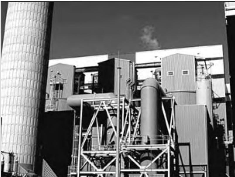
This photo shows the Waste-to-Energy facility's air pollution control devices (including scrubbers, which neutralize acid gases and control mercury), and baghouses, (which remove particulate matter) as well as the continuous emission monitoring system (CEMS).
