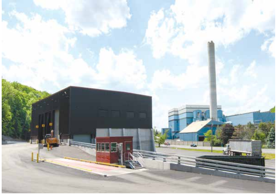
Rock Cut Road Transfer Station in Jamesville is located near the Waste-to-Energy Facility for efficient waste disposal. The WTE is operating at its permitted capacity, though the population is expected to grow soon.
