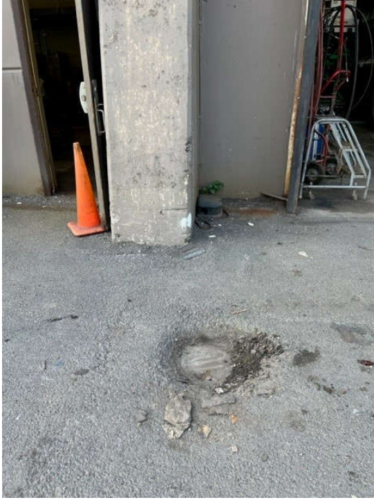
Photo 1: North Site Area, drain cleanout
