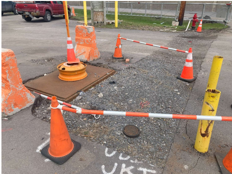
Photo 3: North Site Area, electrical vault cover, utility relocation area, bollards
