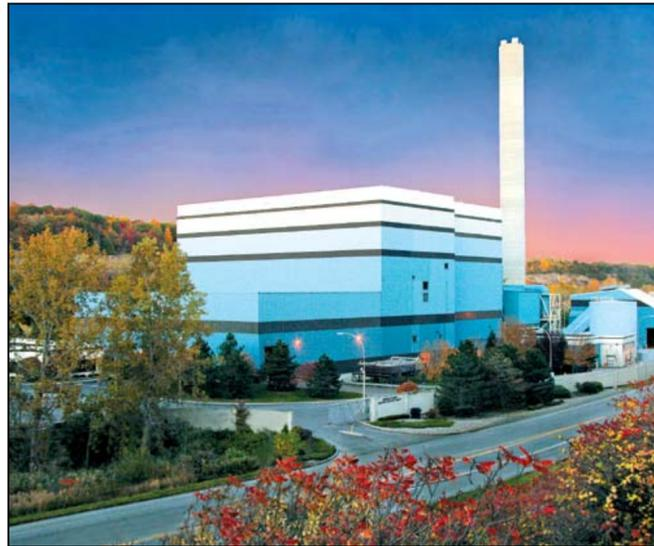
Onondaga County trash is sent to the local Waste-to-Energy Facility where it is burned at 2000°F and converted into electricity (enough to power 15% of homes in our County), all while staying well-below NYSDEC permit limits.
