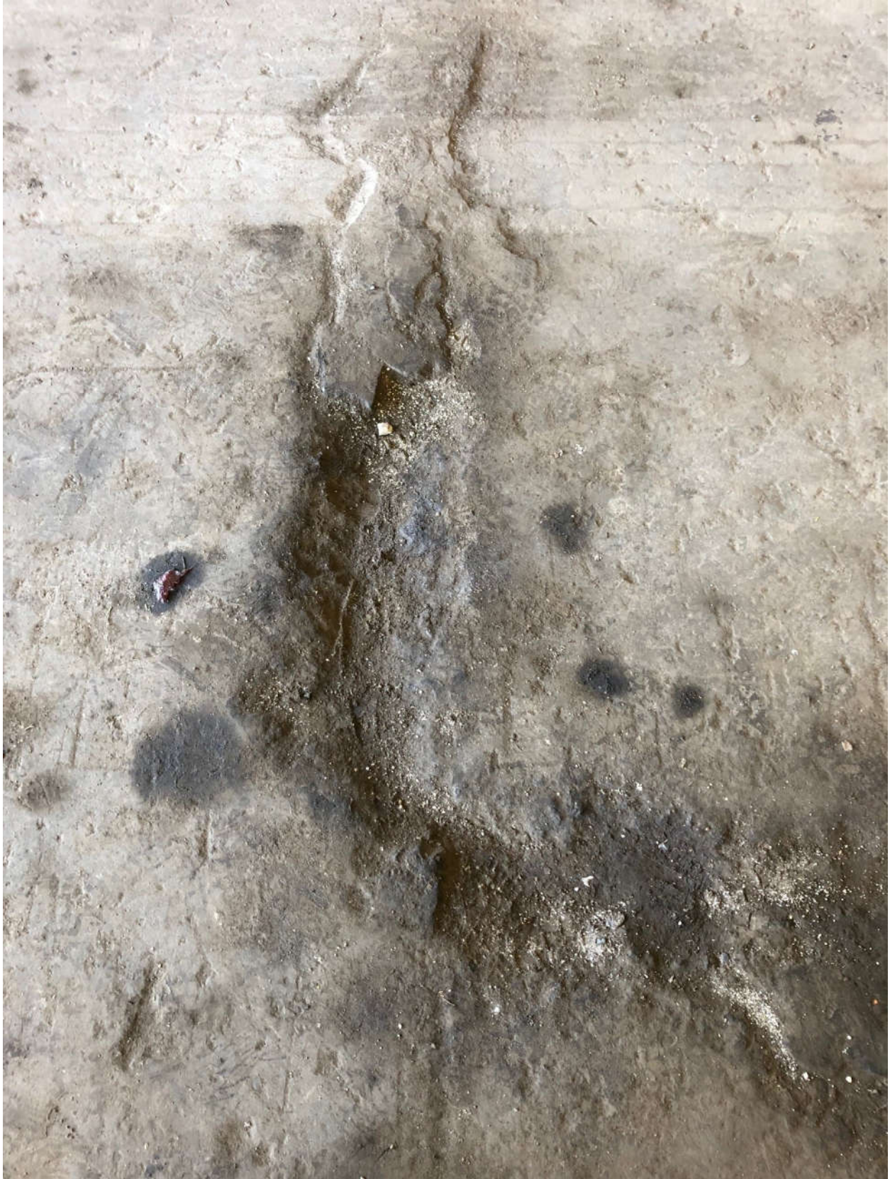
Damaged floor section
