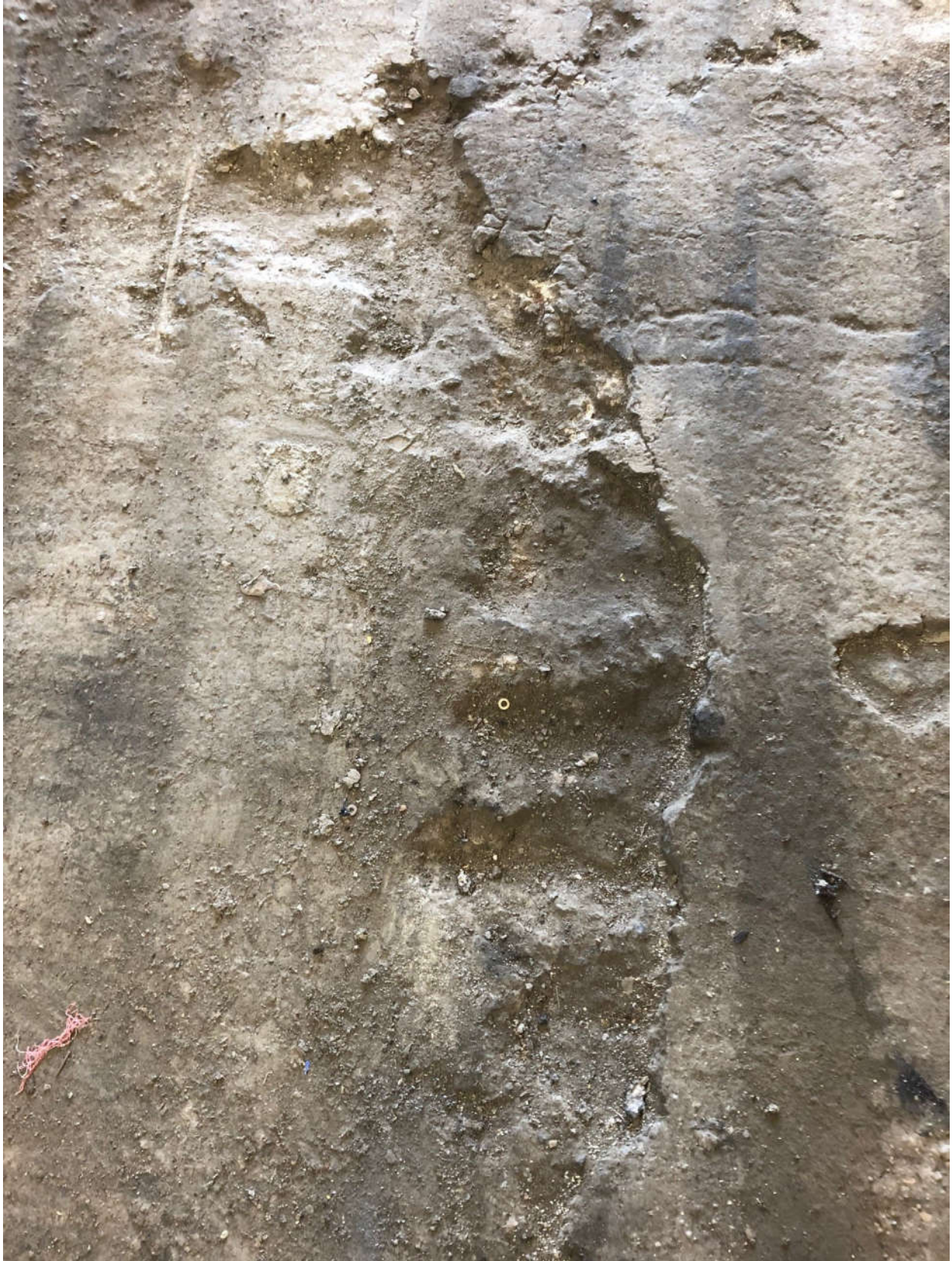
Damaged floor section
