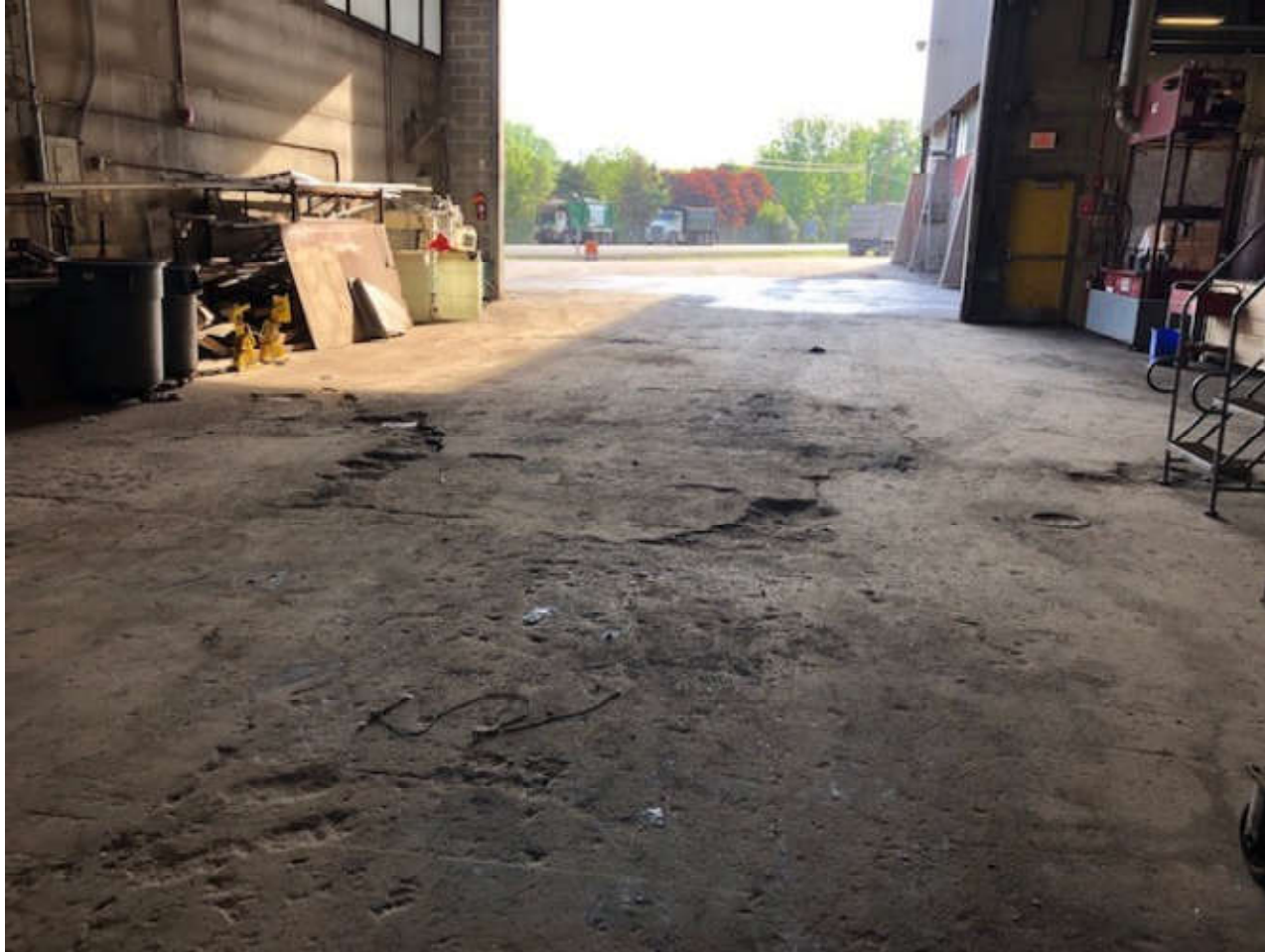
Facing East. Building 1 Long Bay Damaged Concrete
