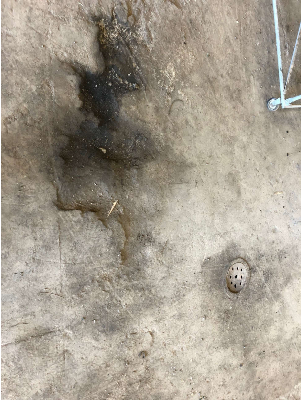
Damaged floor with approximate location to floor drain
