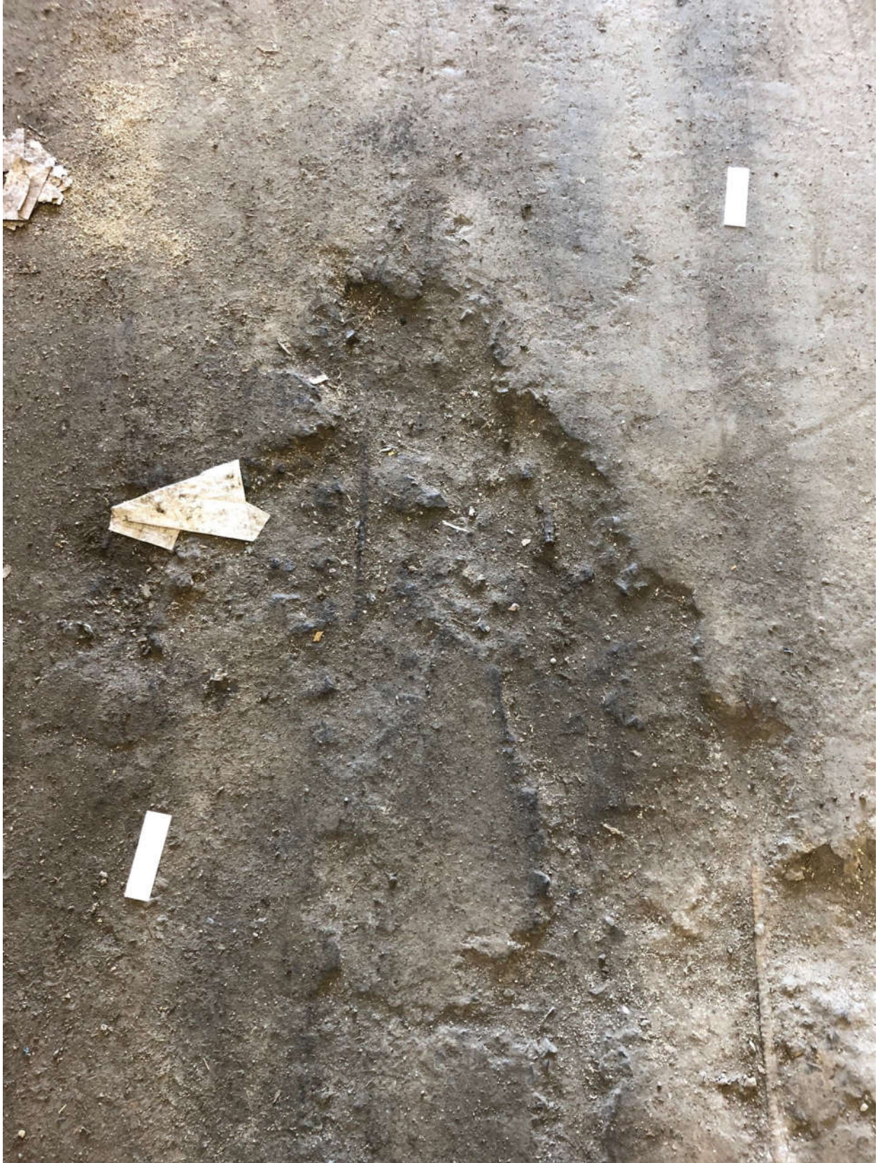
Damaged floor with exposed rebar
