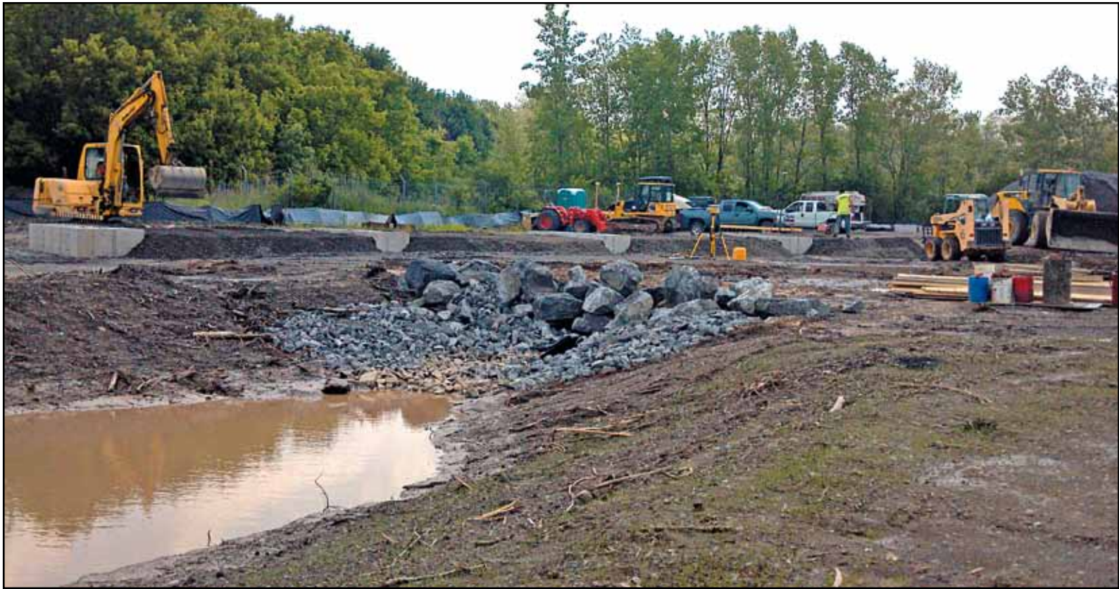
Amboy Compost Site upgrades include a new entrance road, a permanent scale, a new concrete aeration pad, a fabric receiving building, a storm-water retention pond, an office trailer, and an enhanced residential use area. The storm-water retention pond, which protects water quality, is shown here.
